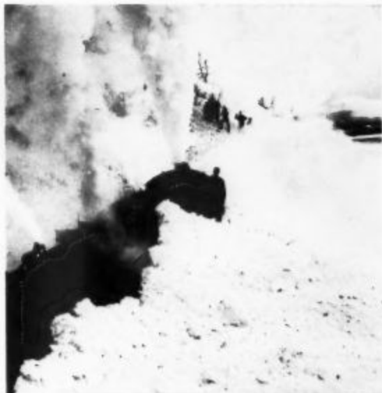
... bulldozers, which scraped a trail along the top, and a . . . . . 125-ton rotary plow pushed by two 2-8-0 steam locomotives
