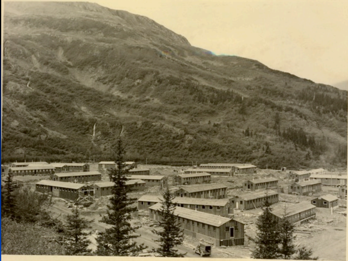
1943 Original wood frame garrison construction
