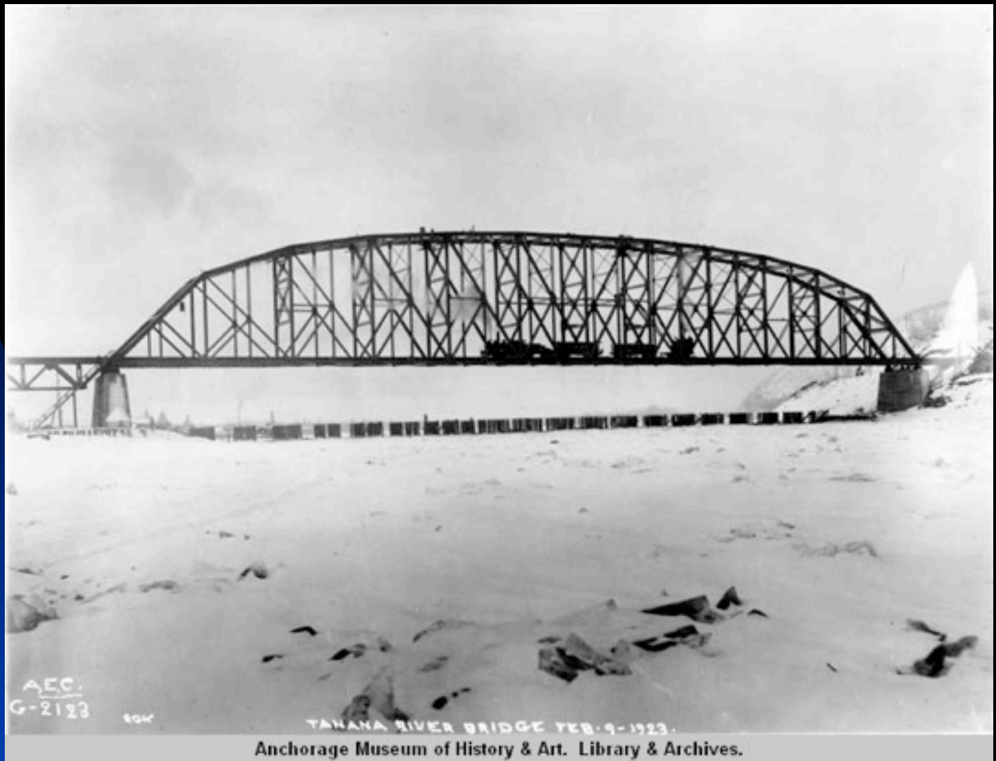
Feb 9, 1923 First train over the Tanana River Bridge. At 704 ft. the world's longest single span bridge.
