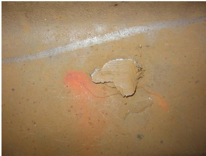
Figure 42: Web Defect Developing from Bond Application
