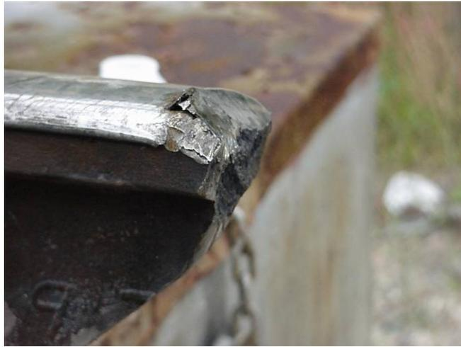
Figure 11: Impact Batter from Rolling Stock Wheels
