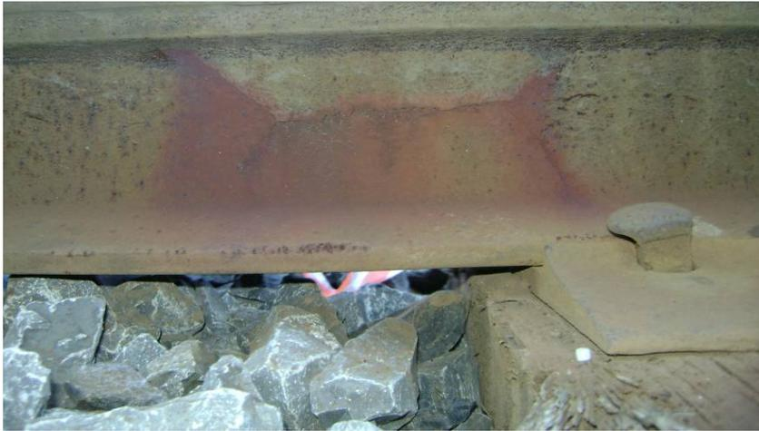
Figure 30: Split Web Defect Showing Bleeding Condition Along Crack Development
