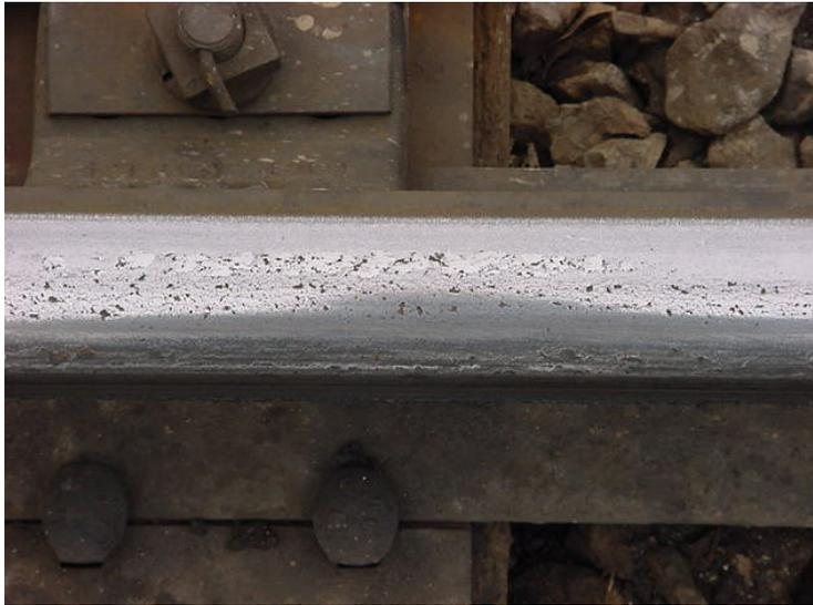
Figure 48: Centralized Flaking Condition Showing Chipping of Parent Metal
